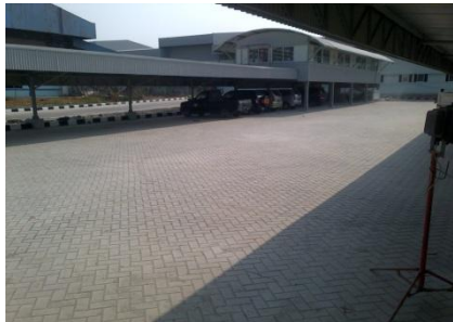
Project Paving Car Port PT. Gajah Tunggal, Tangerang
